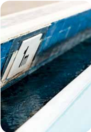
Below deck, recessed gutter made from steel reinforced concrete
