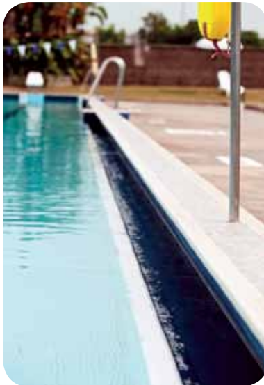
Below deck, recessed gutter made from steel reinforced concrete
