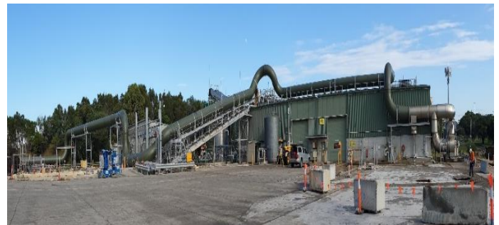
Figure 2 Installed ventilation ductwork on biosolids building and area where biofilter previously was
