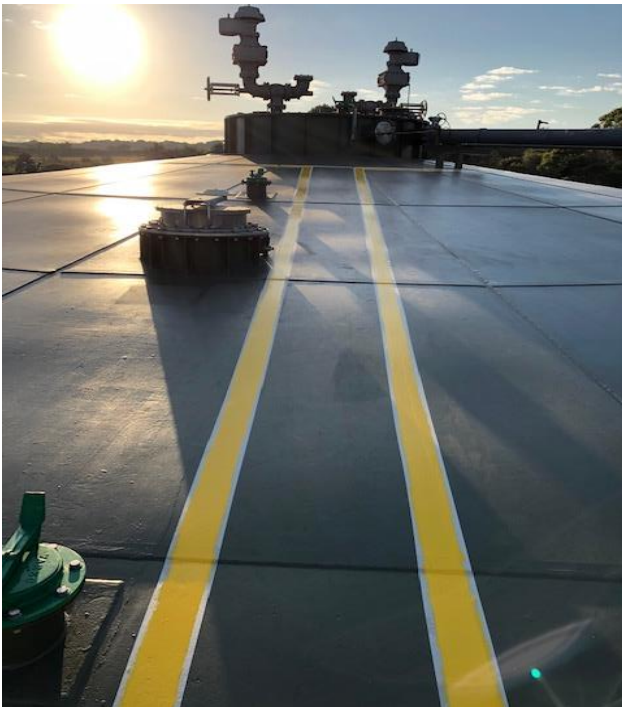
Figure 1 Refurbished roof of cleaned and almost finished 3rd digester
