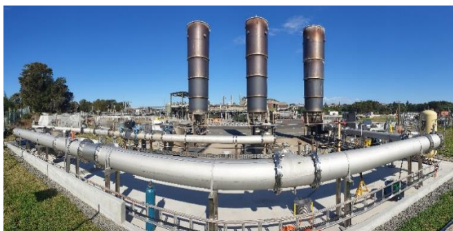
Figure 3 Waste Gas Burner Pipework Upgrades
