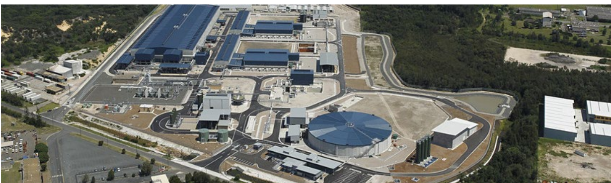
Image: Sydney Desalination Plant
