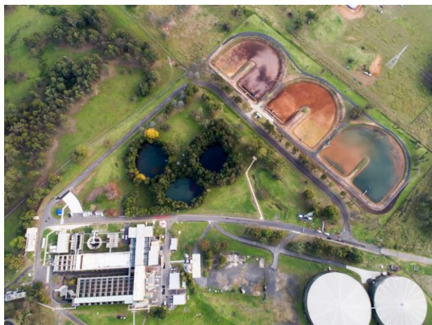
Orchard Hills Water Filtration plant
