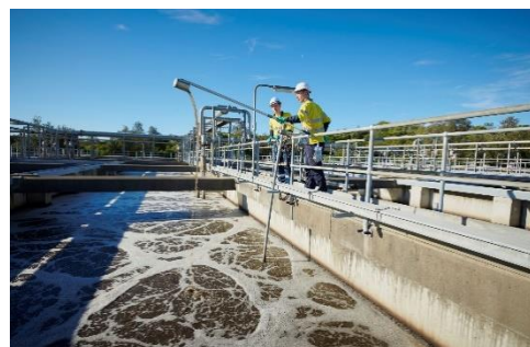
Sampling mixed liquor in aeration phase.
