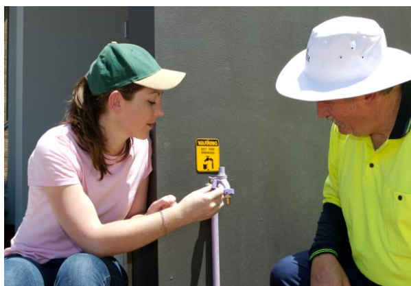
Ensure the recycled water handle is removed when the tap is not in use.
