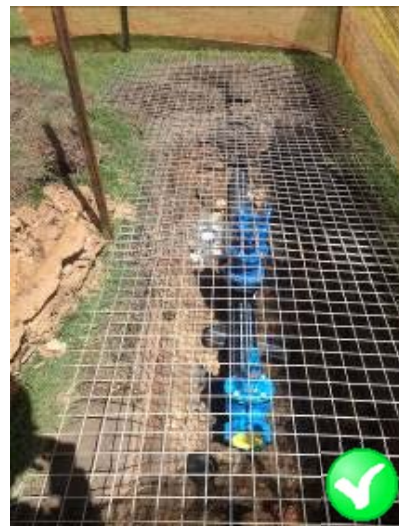
Figure 2 Fittings capped overnight in trench
