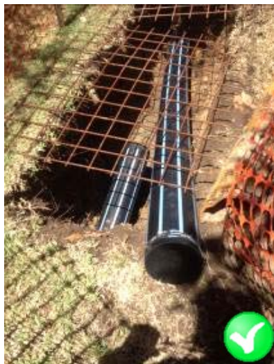
Figure 1 Pipes capped overnight in trench
