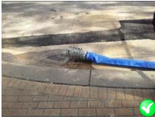
Figure 8 Discharged water directed away from trench
