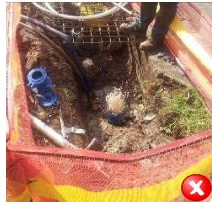
Figure 9 Discharged water into Trench
