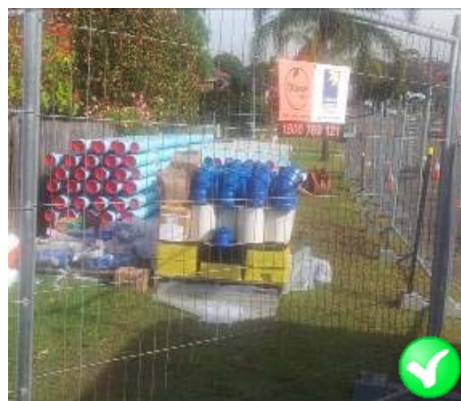
Figure 4 Pipes and fittings stored with protective caps
